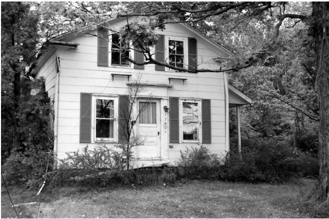
Harvery Hollister house before tear down fall of 2008
