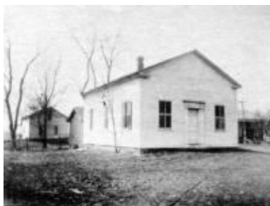
Town Hall—Circa 1914 Now—Burns Lindow Bldg
