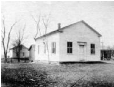
Town Hall—Circa 1914 Now—Burns Lindow Bldg
