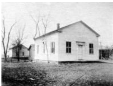
Town Hall—Circa 1914 Now—Burns Lindow Bldg
