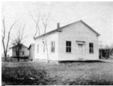
Town Hall—Circa 1914 Now—Burns Lindow Bldg
