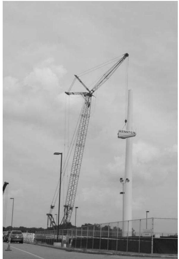
Crane hoisting turbine on tower At Kenston High School
