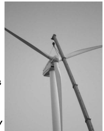
Turbine Blades installed August 28, 2012
