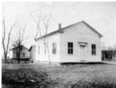
Town Hall—Circa 1914 Now—Burns Lindow Bldg
