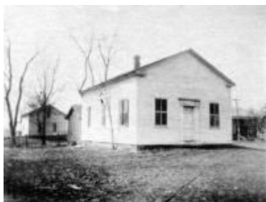
Town Hall—Circa 1914 Now—Burns Lindow Bldg
