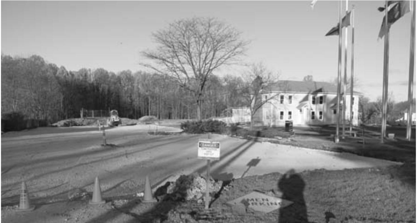
Construction on driveway and parking area to Bissell House November 2011
