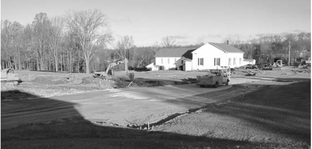
Construction around Bainbridge Town hall November 4th, 2011
