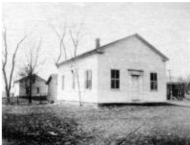
Town Hall—Circa 1914 Now—Burns Lindow Bldg
