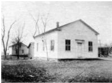
Town Hall—Circa 1914 Now—Burns Lindow Bldg
