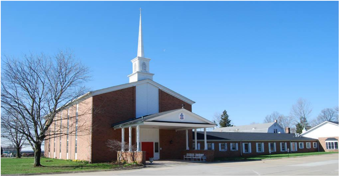
Valley Presbyterian Church today. New church on left with offices to the right connecting to social hall. The top of the old church/gambling hall can be seen on the right behind the church offices. Photo April 2009
