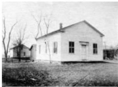
Town Hall—Circa 1914 Now—Burns Lindow Bldg
