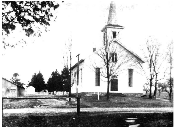
Early view of church with the horse sheds on the left side of church
