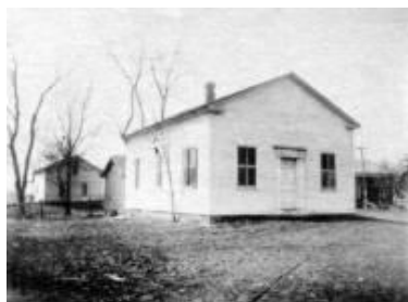
Town Hall—Circa 1914 Now—Burns Lindow Bldg
