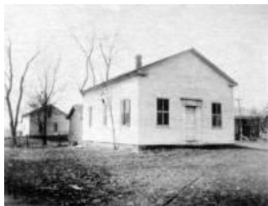
Town Hall—Circa 1914 Now—Burns Lindow Bldg
