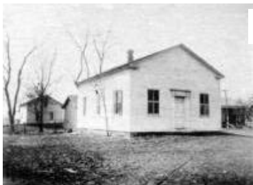
Town Hall—Circa 1914 Now—Burns Lindow Bldg
