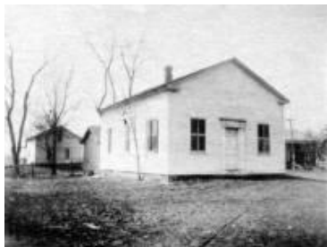
Town Hall—Circa 1914 Now—Burns Lindow Bldg
