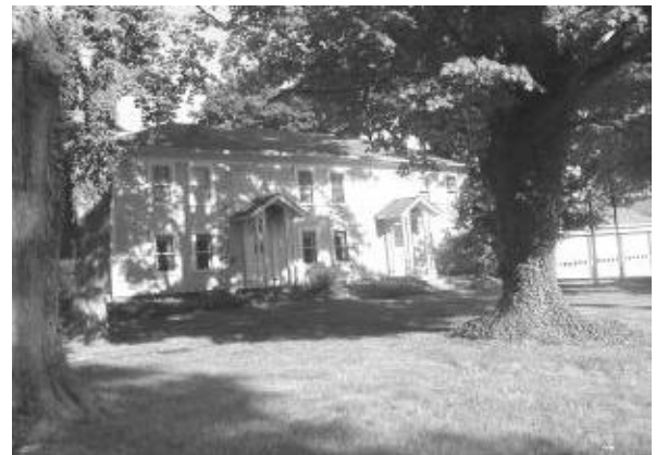
Former Tucek Home purchased by Bainbridge Township. (2002 photo)
